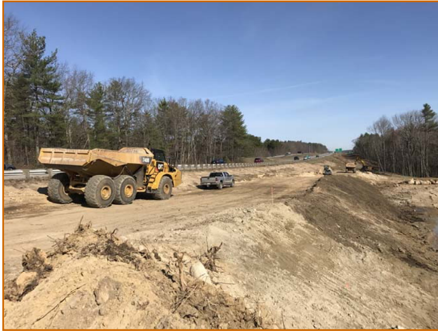
PLACEMENT OF EMBANKMENT ALONG NORTHBOUND BARREL.
