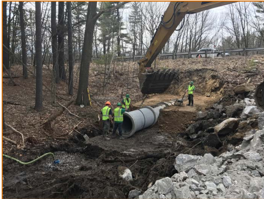
INSTALLATION OF DRAINAGE PIPE EXTENSION ALONG NORTHBOUND.
