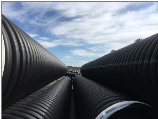
BELOW: PIPES STOCKPILE
