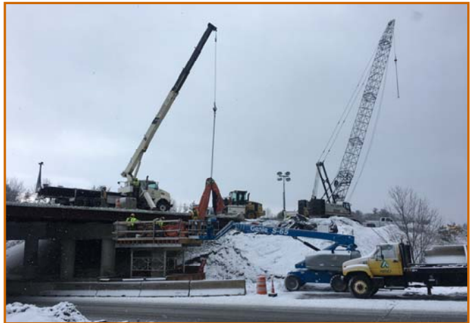
ABOVE: SB NORTH LOWELL ROAD BRIDGE BACK-FILLING
