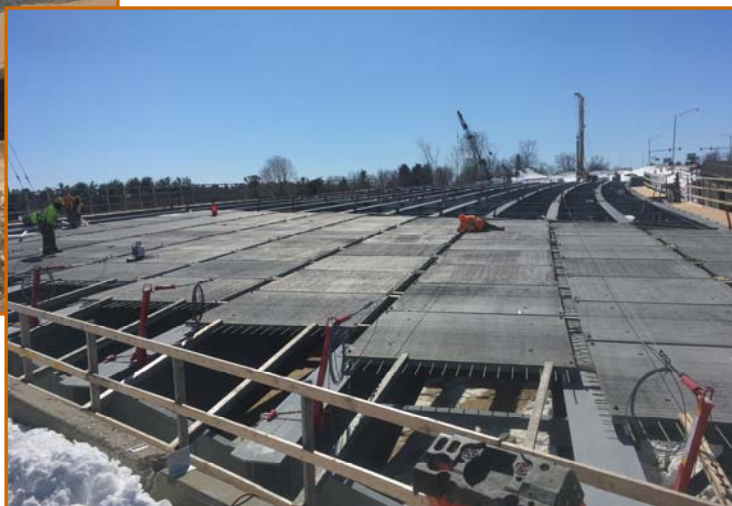
RIGHT: PLACEMENT OF NH ROUTE 102 BRIDGE DECK PANELS
