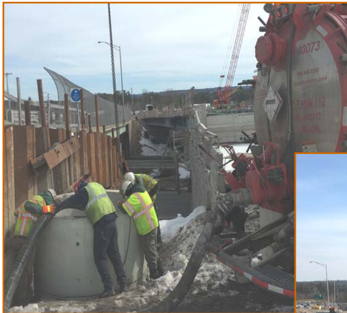
LEFT: VACUUMING OUT THE ROCK SOCKET FOR OVERHEAD SIGN STRUCTURE
