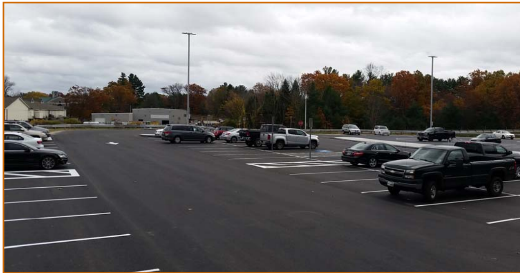
ABOVE: THE NEW EXIT 3 PARK AND RIDE OPENED FOR OPERATION ON NOV. 6, 2017, PROVIDING 140 SPACES FOR VEHICLES.
