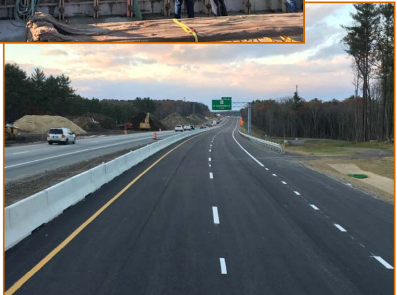
RIGHT: NEW NB BARREL READY TO RECEIVE TRAFFIC, FACING NORTH
