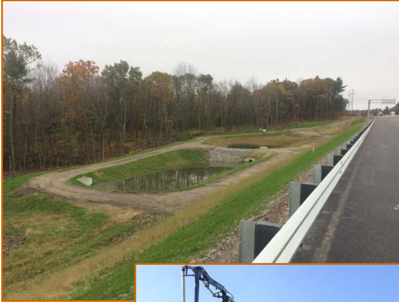
LEFT: DRAINAGE DETENTION BASIN COMPLETED, SEEN FROM FINISHED ROADWAY, FACING SOUTH.
