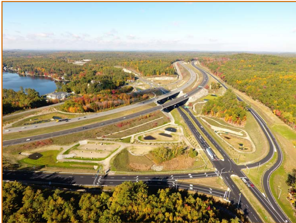
I-93 EXIT 3 AREA IMPROVEMENTS. FACING NORTHWEST. NB OFF-RAMP (LEFT SIDE) AND ON RAMP (RIGHT SIDE) AS IT INTERSECTS NH 111 IN THE FOREGROUND AND I-93 NB & SB IN THE BACKGROUND.
