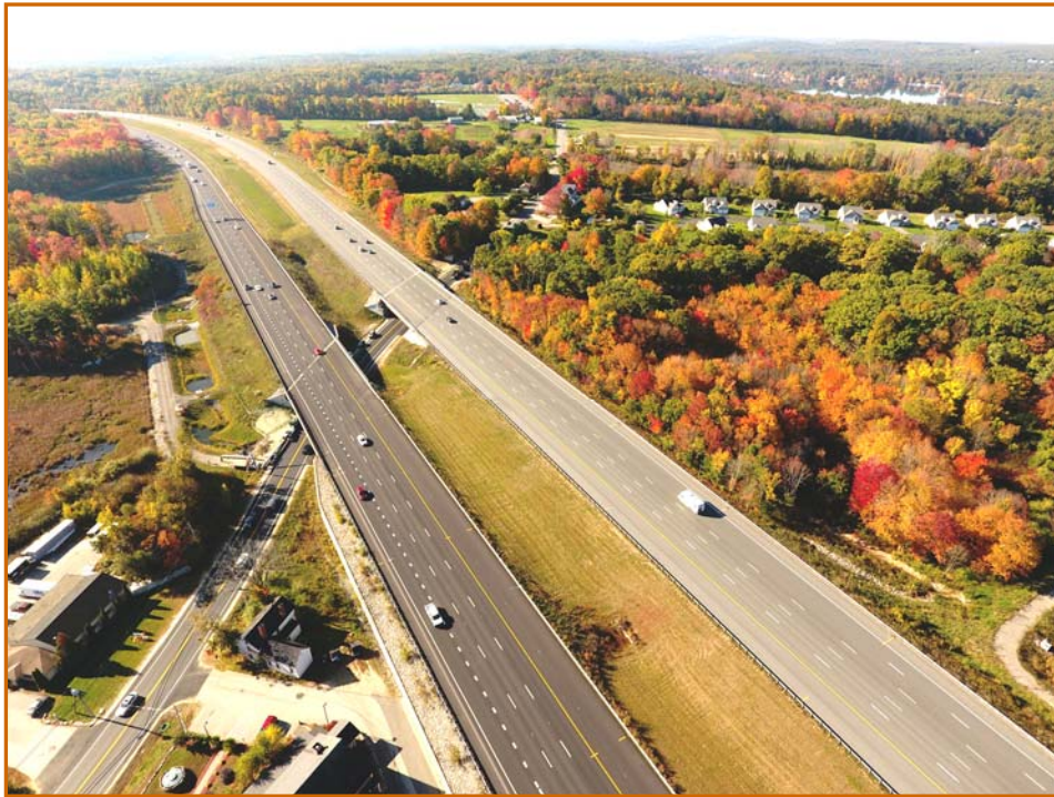
I-93 CROSSING NH 111A. FACING SOUTH.
