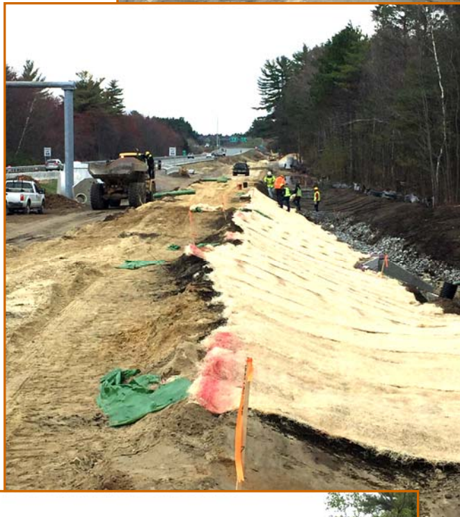
LEFT: STABILIZING BACK SIDE OF SOUNDWALL BERM WITH LANDSCAPE MATTING.
