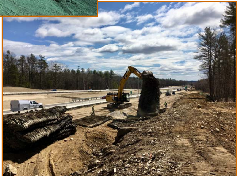
RIGHT: SETTING BLASTING MATS PRIOR TO SB LEDGE BLAST, FACING SOUTH
