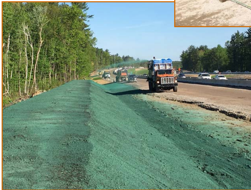
LEFT: I-93 SB SOUNDWALL BERM HYDROSEEDING, FACING NORTH.
