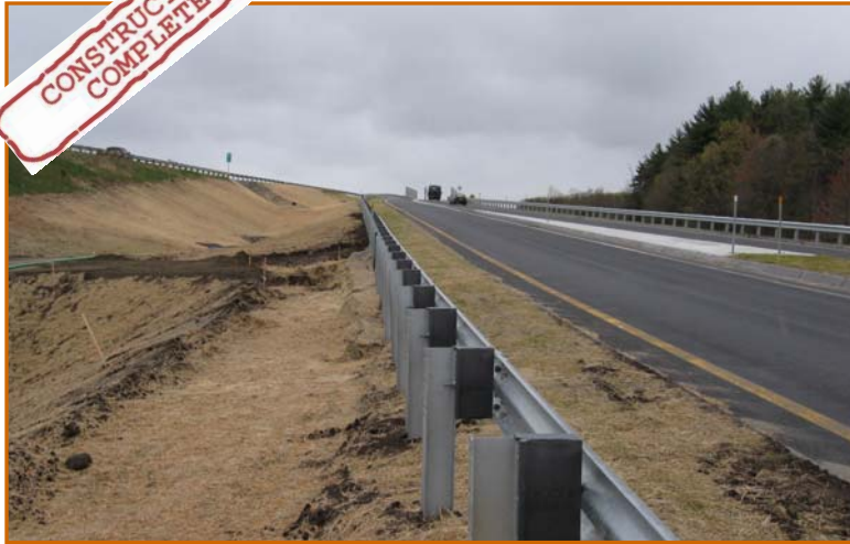
Looking North Along the New NB On-Ramp 04-28-2010
