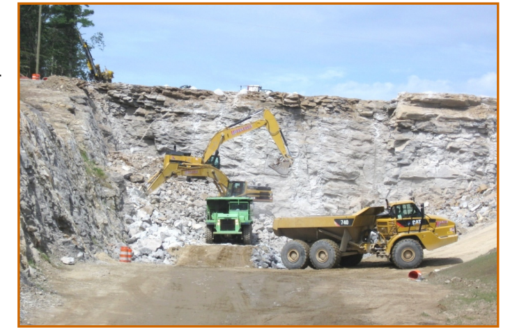
ROCK & LEDGE REMOVAL OPERATIONS
